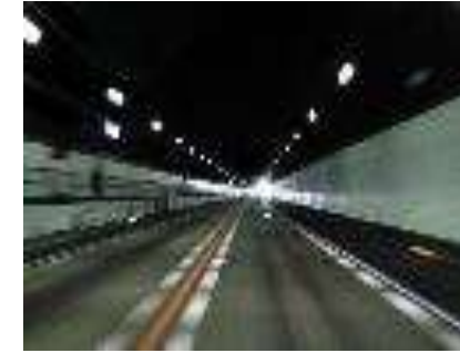
In the highway tunnel for LED lighting
